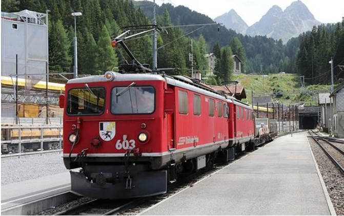
A pair of Rhätische Bahn Ge4/4 I locomotive rests at Preda Aug. 3, 2017, led by veteran No. 603. The existing tunnel is visible at far right; the new construction is hidden by the train.
