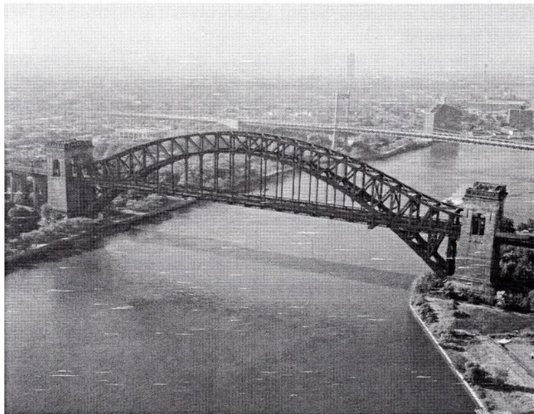
The Hell Gate Bridge has more than 1.17 million rivets, according to photographer Dave Frieder. (Photo: Jet Lowe, via Library of Congress)
