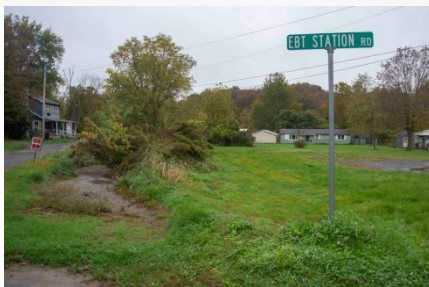
"EBT Station" street sign in Saltillo, Pa., may be prophetic in light of a Friends of East Broad Top campaign to rebuild the town’s station. The gray area to the right of the sign is the former station location; tracks still exist between the sign and station site but are hidden by the grass. (Dan Cupper) Right: Mixed train stops at Saltillo in 1952. (Philip R. Hastings)
