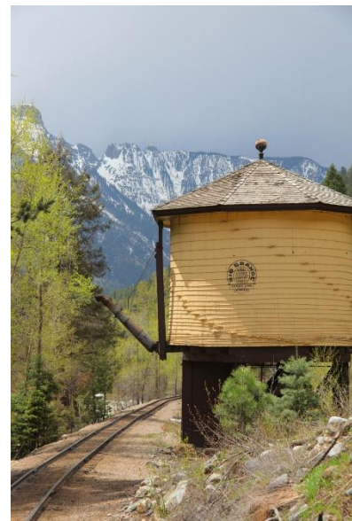
One of several water towers along the way.
