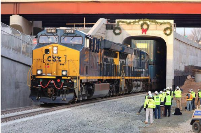
CSX Transportation ET44AH No. 3319 emerges from the newly completed Virginia Avenue Tunnel with double stack containers in tow. The train is in route to North Baltimore, Ohio, from Portsmouth, Va., along the route of CSX Transportation's National Gateway project.
