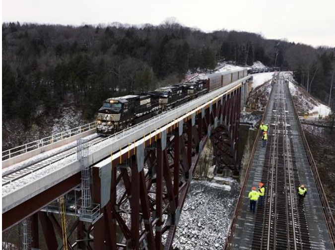
Norfolk Southern C44-9W No. 9345 leads train 36T, a Buffalo, N.Y., to Allentown, Pa., manifest train on a new steel arch span on Dec. 11. The arch replaces an iron truss bridge built by the Erie Railroad in 1875 and shown on the right.
