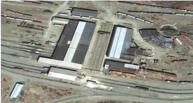
New England has a major new facility for the cleaning, repair, and fleet management of tank cars.
