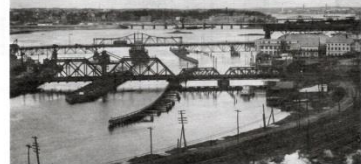
A view of the Seekonk River with its moveable bridges, from East Providence looking north toward Pawtucket in the distance. In its down position, the Crook Point Bascule Bridge is at top center. In the foreground is the India Point Railroad Bridge, a swivel bridge near the Brown bathhouse. The swivel portion has been dismantled and removed although the stationary portion on the right remains today. At center, a trolley is seen crossing the Seekonk River towards East Providence. This swing bridge predates the Washington Bridge, a bascule drawbridge that opened in 1930. At top right distance, the old Red Bridge, another swing bridge, is visible. It was dismantled in 1966 and later replaced by the Henderson Bridge, a stationary bridge sometimes also known as the Red Bridge. (The Providence Journal files)
