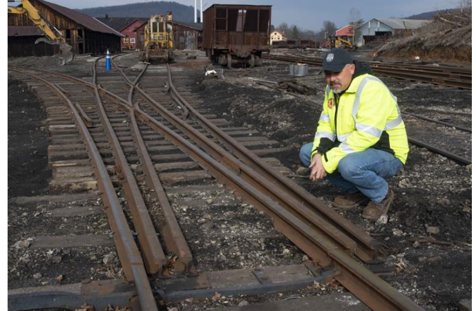
East Broad Top General Manager Brad Esposito looks over a recently rehabilitated three-way stub switch at the south end of Rockhill Furnace Yard.
