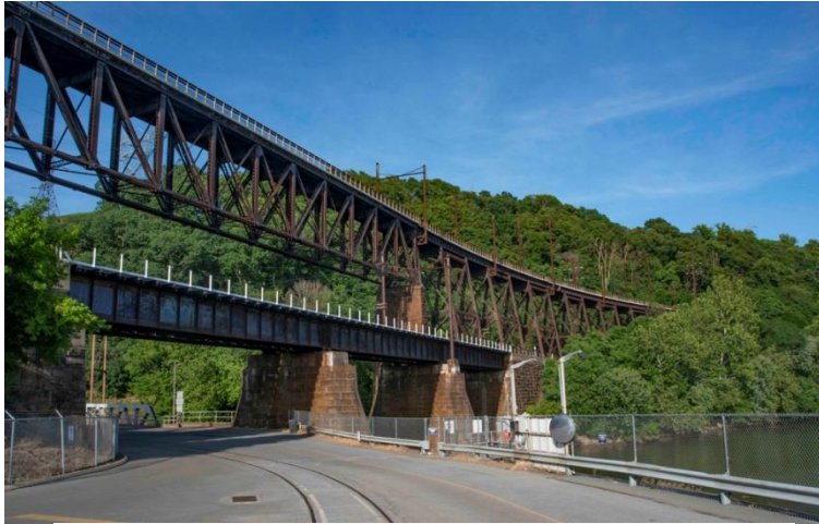
The 150-foot-high Safe Harbor (Pa.) Bridge, has been repurposed for public trail access. The lower bridge carries Norfolk Southern's still-active Port Road Branch. (Dan Copper)
